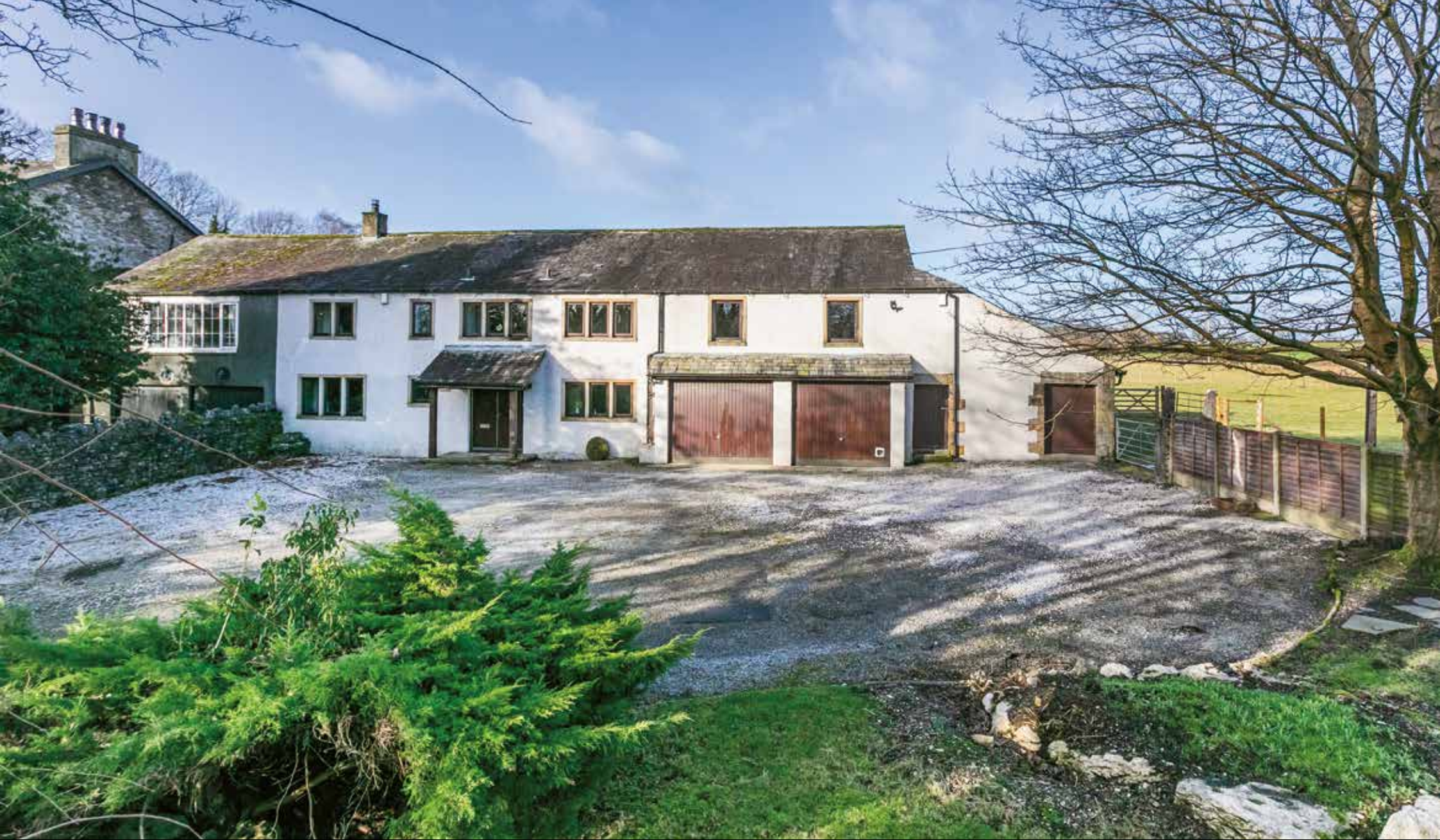
Dale House Barn Tewitfield | Lancashire | LA6 1JH
