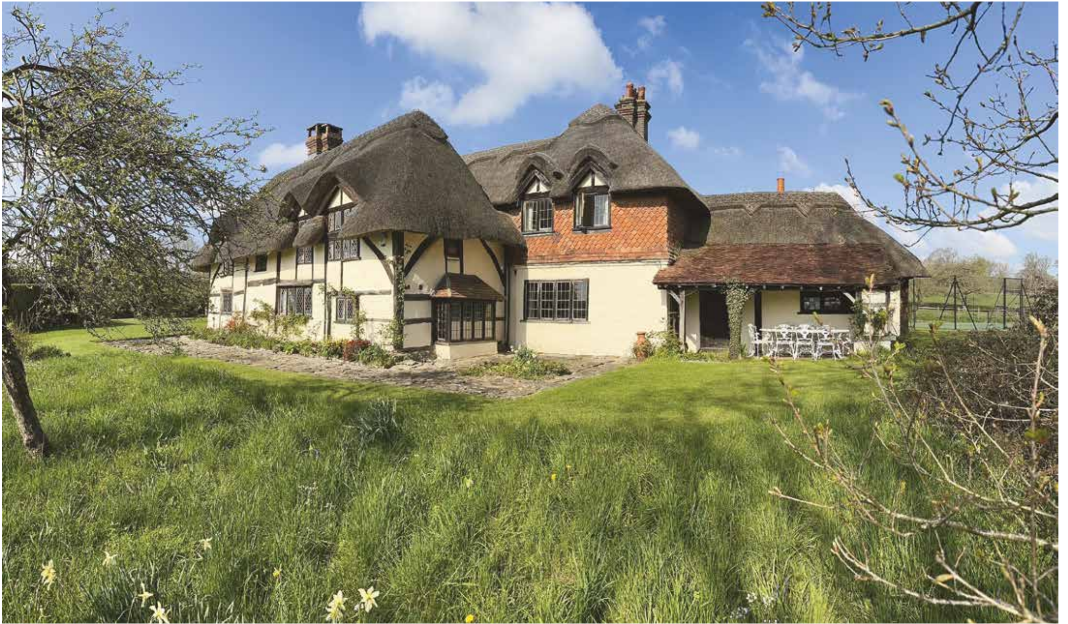
Dormer Cottage Stan Hill | Charlwood | Surrey | RH6 0EP
